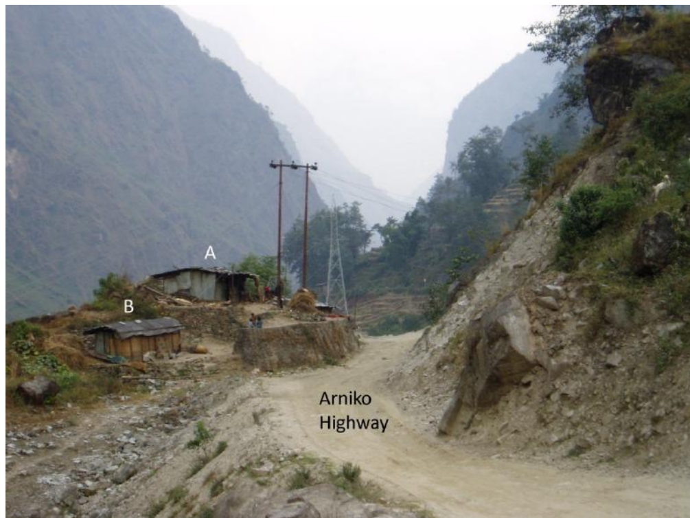
Figure 4.14 “4 km Settlement”. The house (A) was originally located where the goat shed is now (B) but was destroyed by a falling boulder in 2006. The strategic road linking Kathmandu and China (Tibet) is frequently blocked by landslides.
