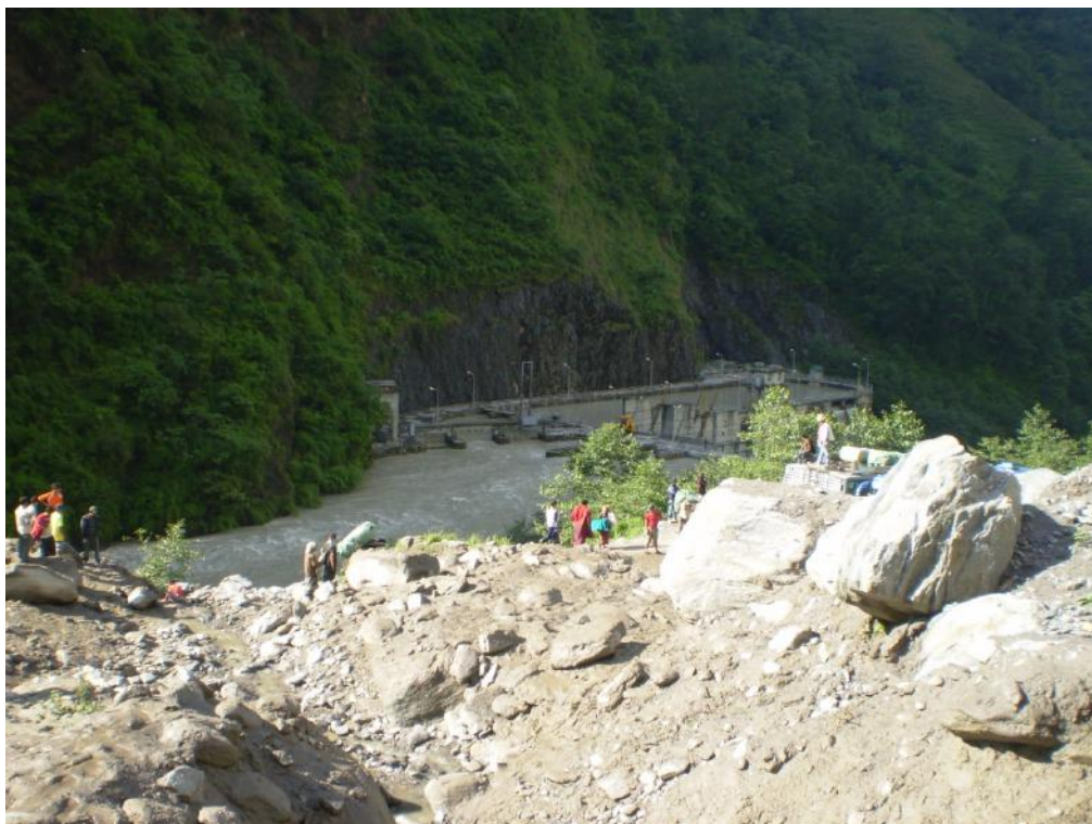
Figure 4.17 The Tatopani debris flow reactivated following heavy monsoon rains in July 2007. Landslide material partially blocks the Bhoté Koshi River behind the Tatopani hydropower dam.
