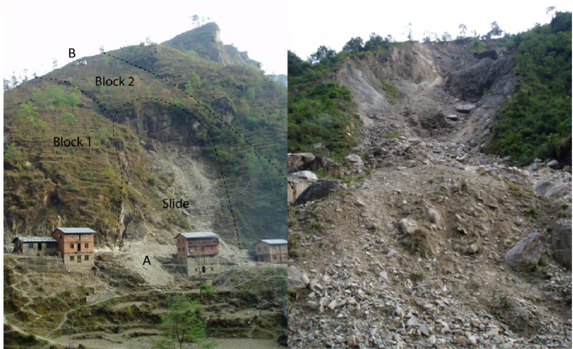
Figure 4.12 Left - The active translational slide in Chaku. Five houses were destroyed by a landslide in 2001 (A). A house remains occupied above the main scarp of the landslide (B) which is retrogressing up the hillslope putting more houses at risk. Right – A colluvial fan at the bottom of Chaku settlement. Evidence of secondary lateral slumping can be seen.
